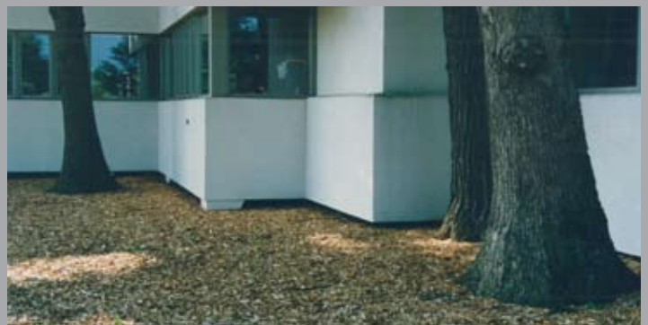
The whole structure is supported above ground level by foundation pads, which caused relatively little damage to roots and the rooting environment.
