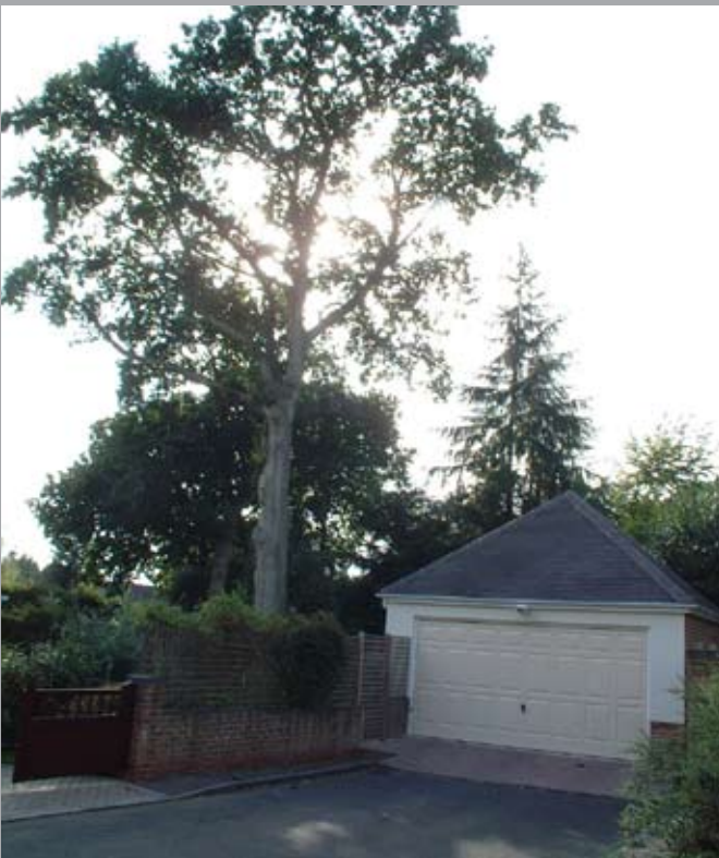
The completed garage and tree in 2002.
