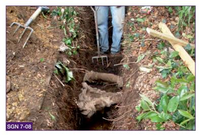
Where roots to be retained will be exposed for longer than a few hours and there is a risk of drying out, the hessian covering should be kept damp by watering.
