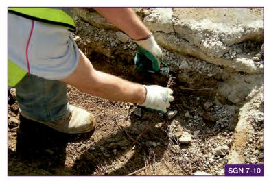
Where roots have to be removed, they should be cut cleanly beyond the face of the excavation with secateurs or a saw.
