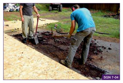
Conventional hand tools such as spades and forks should be used where surfacing is so hard and compacted that it is not possible to use air tools.
