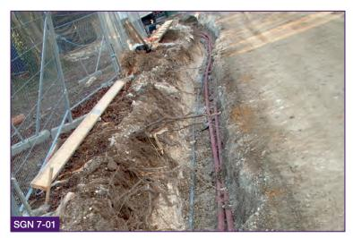
All excavation in RPAs should be with hand-held tools. Where possible, there will be a preference to use air tools because they are very effective at exposing roots and services with minimal damage.
