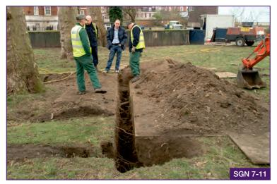
Where large amounts of soil are excavated to expose roots, it should be temporarily stored on heavy duty plywood boards, or similar, to prevent ground compaction to the RPA beneath.
