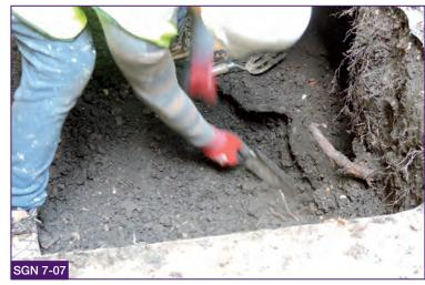
Exposed roots to be retained should be protected from light, drying out, and extremes of temperature, by covering with hessian sacking and/or boards until they can be covered back with soil.
