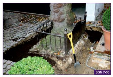
These cobbles and the subsurface were so compacted that hand tools had to be used to loosen and then remove the material around the roots before replacing with a more favourable rooting medium.
