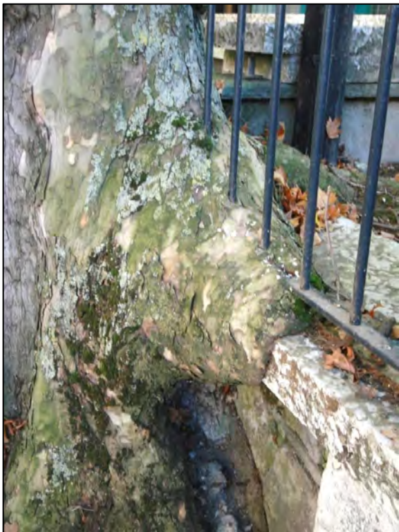
Photo 4: Root and trunk growth will deform around robust structures if the forces required to move them are too great (Geneva)
