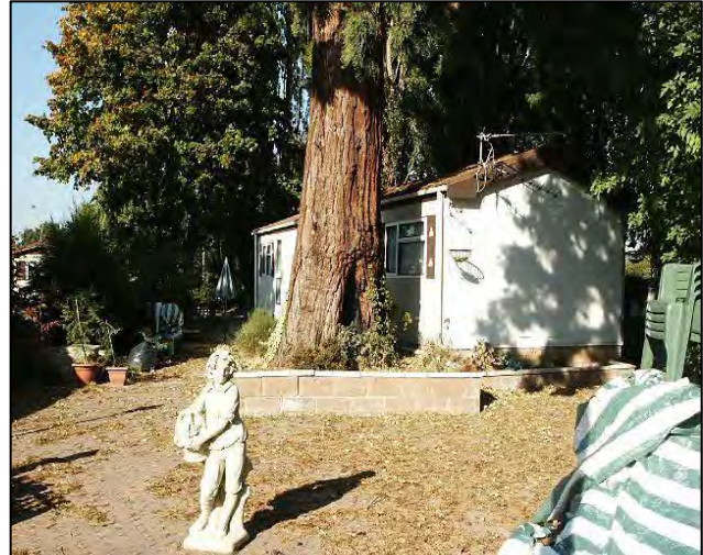
Photo 6: The potential for damage to this light structure from both root growth and transmission of trunk movements is obvious (UK)
