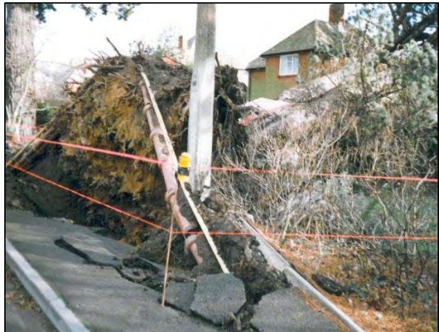
Photo 7: This 25m Monterey pine blew down in the 1990 storms, bringing up the pavement and services with its massive root ball (Ferndown, Dorset)
