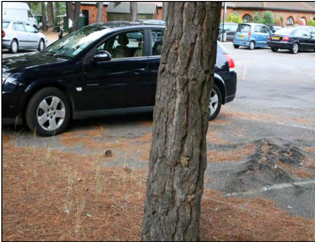
Photo 2: Root growth from this young Monterey pine has severely disrupted car park surfacing (Ferndown, Dorset)
