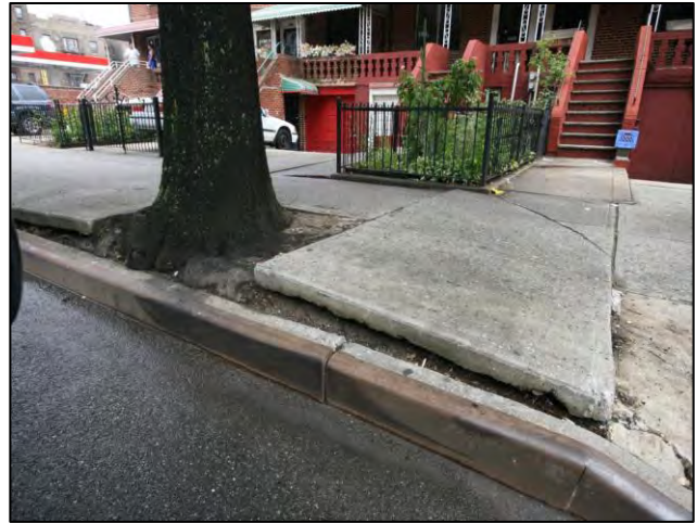
Photo 3: Pavements and sidewalks all over the world are susceptible to lifting from root growth (New York)
