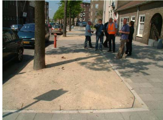
Henk Werner (Pius Floris tree experts) in the fluorescent jacket describes the combination of root pruning and root deflector installation on mature trees causing surface disruption. Ideally, all the surfacing within about 7–10 times the trunk radius is removed. Any roots protruding above the surface are carefully cut and all the roots close to the surface at the outer edge are cut. The root deflector is installed (thin black line around the paved boundary) and a permeable granular finish applied with gradual undulations rather than abrupt trip hazards. With the right level of aftercare, Henk has found this a very successful strategy for prolonging the useful life expectancy of larger trees and it is mainstream practice in Amsterdam.
