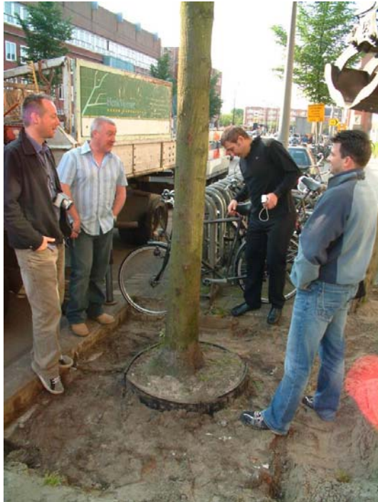
Steve Chatwin-Grindey, Director of DeepRoot UK, removes one section of the deflector to reveal the solid woody roots inside in stark contrast to the absence of large surface roots outside.
