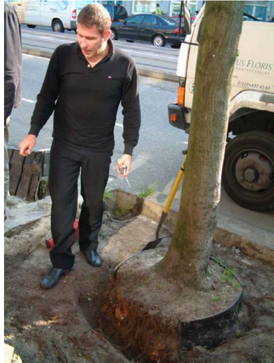
Steve Chatwin-Grindey, Director of DeepRoot UK, removes one section of the deflector to reveal the solid woody roots inside in stark contrast to the absence of large surface roots outside.
