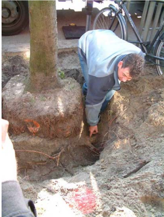
With the DeepRoot deflectors completely removed, Mark Wadey points out one of the structural roots emerging from the rootball about 40cm below the surface.
