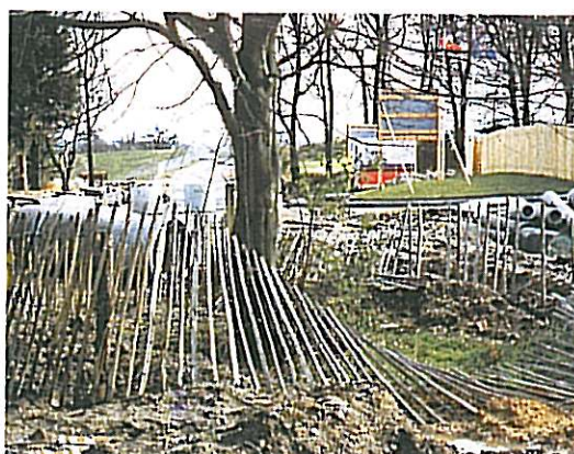
Below left: Board fencing is effective on this Compton Developments site in Poole, while chestnut piling (below) is not.
