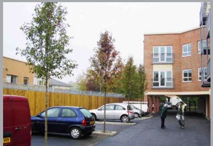
The new surfacing was installed on top of the tree soil and the trees begin to fulfil their planned landscape-softening role with very little loss of parking space. They will also provide much welcomed shade to the parked cars in the heat of summer.
