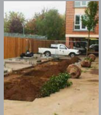
The four new root-balled trees were planted into the planting pits that lined up with landscaping strips between the parking bays.
