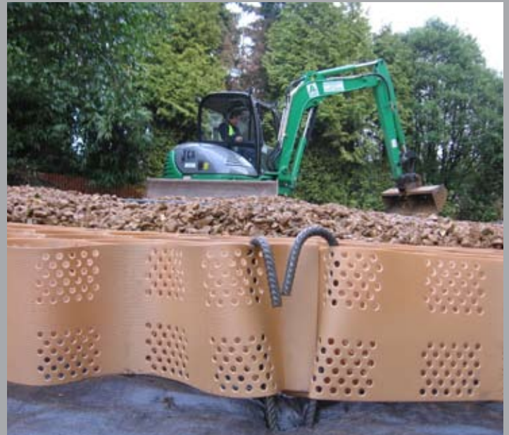
The cells have side perforations to allow the movement of water and air.
