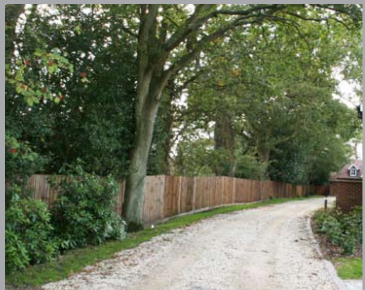
In contrast, using a cellular confinement system filled with stone installed directly onto the ground surface without any excavation often has no significant impact on nearby trees.
