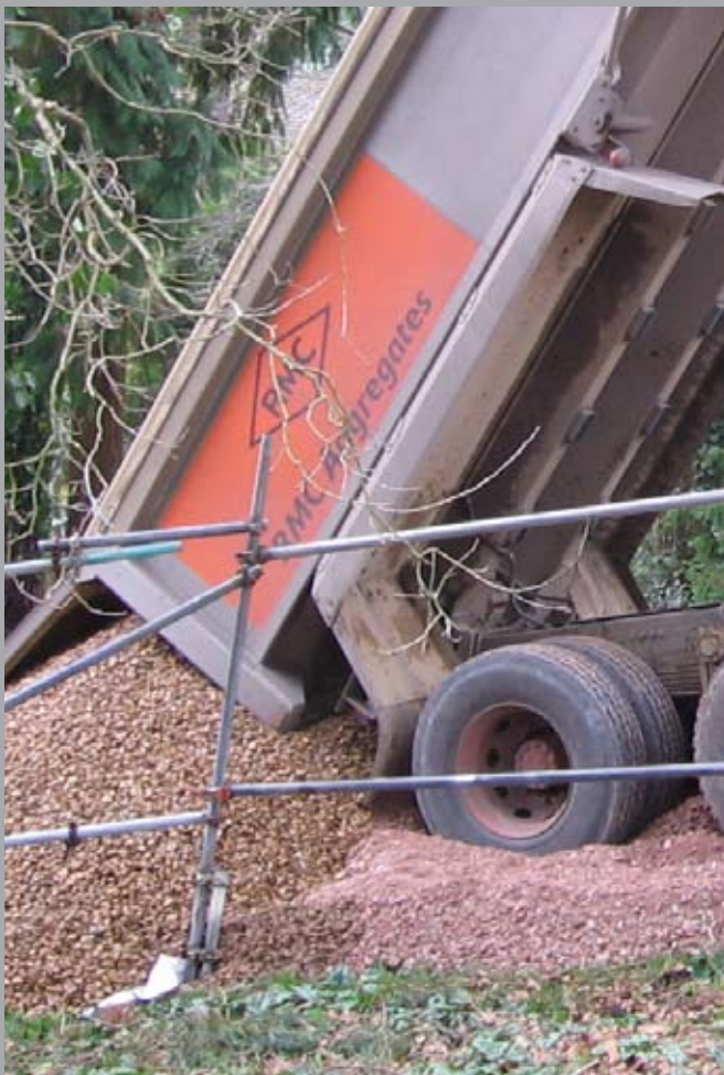
The rigid array of cells can effectively spread the weight of a loaded lorry as soon as they are filled.
